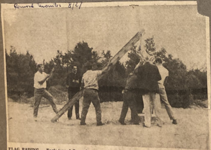
FLAG RAISING — Eagle-topped flag pole at Salvation of Youth home, Pine Haven, is raised by construction workers with help from Father Netto, director of school. Father Netto said construction will be completed shortly and dedication ceremonies are set for Sept. 29. Twenty-two youngsters have been enrolled for this year.
