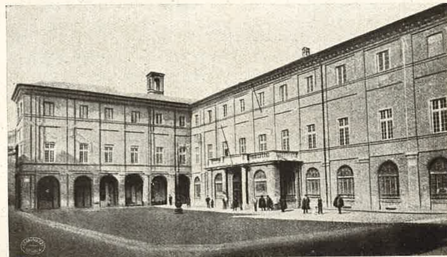
COLLEGIO SAN GIORGIO IN NOVI LIGURE
